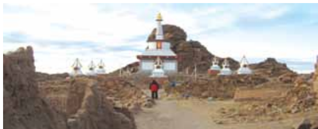
Figure 8.4 Restored Main Stupa at Demchig Monastery Ruins, Khanbogd Soum
